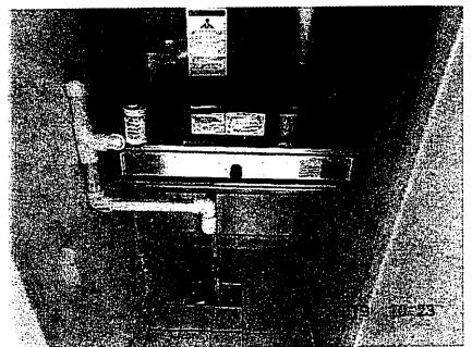
z. **Seal, patch and paint inside the air-handling closet before installing equipment. Seal all air leaks in the supply and return air plenums, adhere to FPL's standards for duct repairs.**
