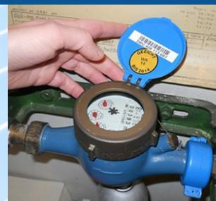
**STEP 2:** Locate where the water pipe enters the building or home. The water pipe should be a one (1) inch wide (i.e., 1-inch diameter) pipe coming from either underground or through the foundation floor or wall.
