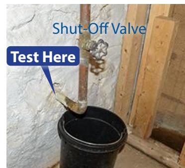
**STEP 4:** Determine what your service line is made of. Water pipes can be plastic, copper, galvanized metal, or lead. First, visually inspect the test area on your water pipe. You may need to rub off any paint, corrosion, or buildup on the outside of the pipe to get a good look. Compare your pipe to the chart below:
