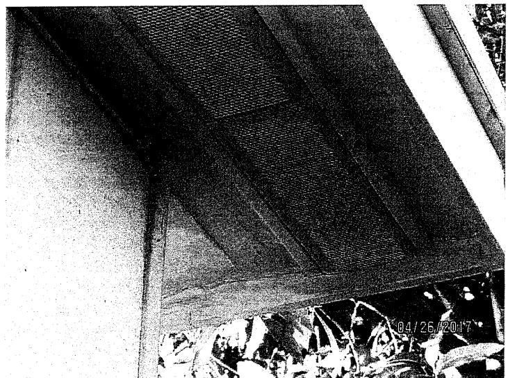
and soffit removed, after fascia and soffit replacement. Paint replaced fascia and soffit, per the General Paint Specifications, to match existing, providing a uniform opaque coverage.
